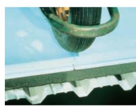
STYROFOAM DECKMATE over metal roof-deck
